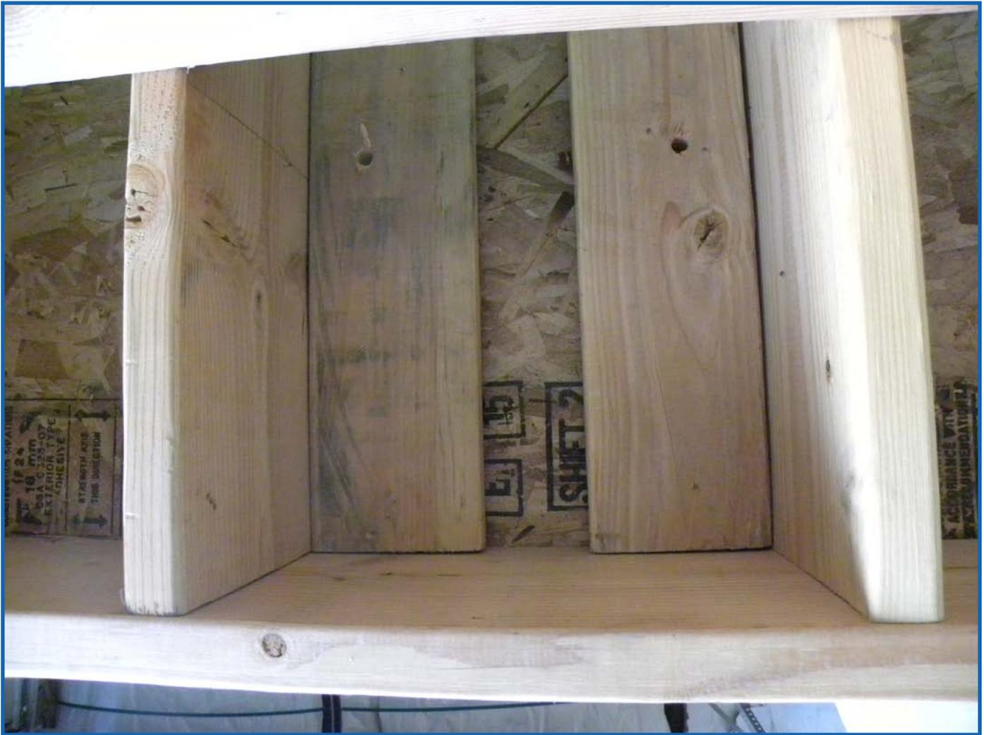
**REINFORCING BOARDS: INSTALL AGAINST FLOOR JOISTS AND FRONT PLATE
