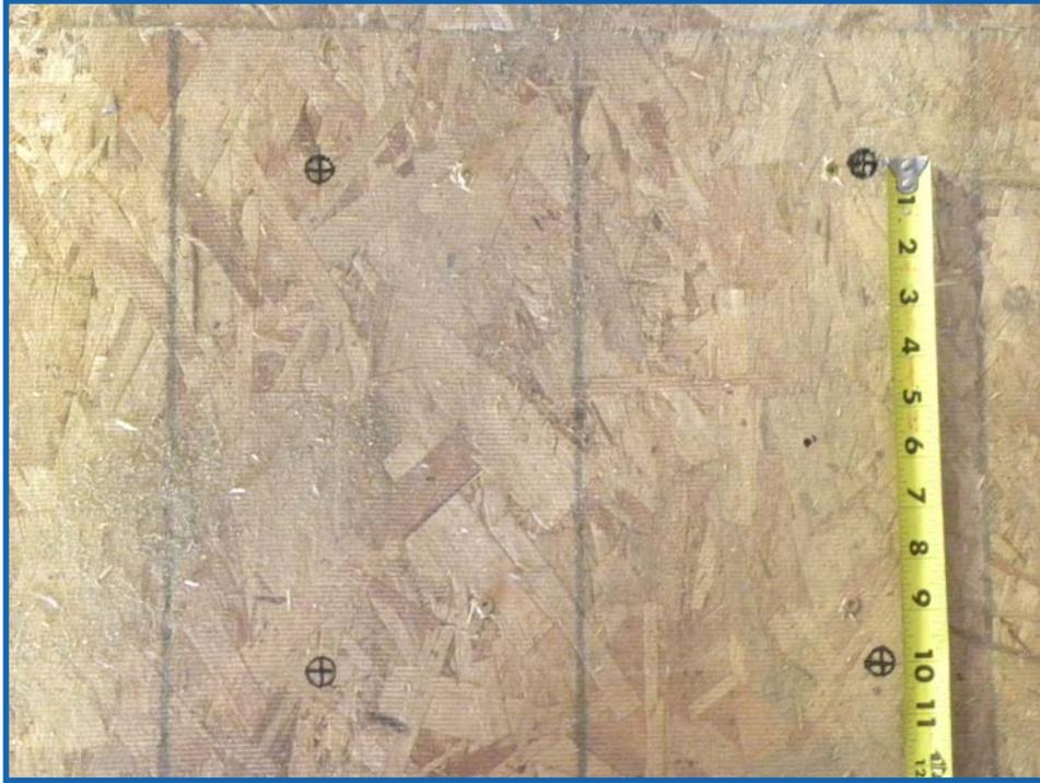
**HINT: USE A TAPE-MEASURE TO CHECK THE HOLES ARE 11" x 10" SQUARE**
