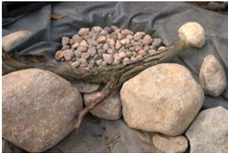
The gravel will also provide a suitable base for leveling the Waterfall Spillway. The Waterfall Spillway should be level from side to side and tilt forward a ¼ bubble on a 2 foot level.
