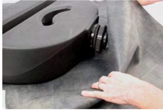
Step 4. Using a screw driver or awl, puncture a small hole in the liner through the center of the Waterfall Spillway fitting. This will be your reference point for the location of the liner connection.
