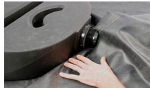
Step 8. Place the second rubber gasket onto the fitting. Note: The liner should be located between both rubber gaskets.
