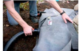
Step 11. The joints around the face of the Waterfall Spillway and surrounding waterfall stones can now be filled with Aquascape Black Waterfall Foam. The waterfall can be operated once the foam is dry.
