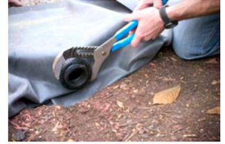
Step 10. Install the included pipe fitting into the back of the Waterfall Spillway. Use Teflon tape or silicone sealant (not included) on the threads of the fitting, in order to provide a water tight seal. Be careful to not over tighten pipe fitting, which could possibly crack the plastic fittings. The filter is now ready for the pipe to be installed.
