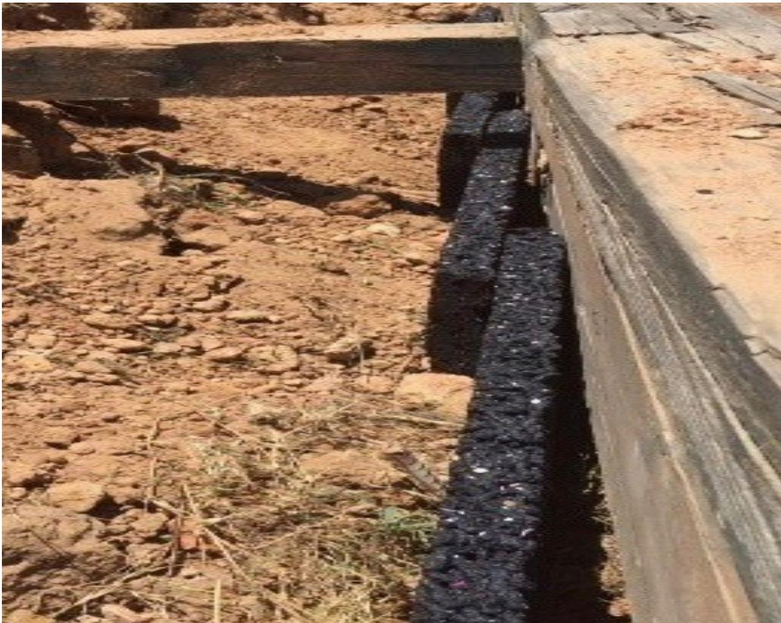
**HydroBlox** provides a high-load strength, puncture-resistant layer for retaining walls that can improve drainage, stabilization, and stormwater management. Compatible with either hard or soft landscaping, HydroPlanks quickly pull water out of the retaining walls and keep the structure from becoming too saturated and collapsing. Lay out the planks end to end, and side by side, and place the backfill directly onto the HydroPlanks.
