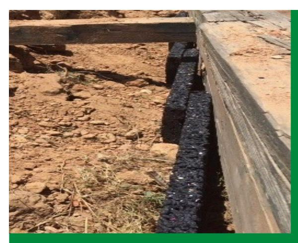
**HydroBlox** provides a high-load strength, puncture-resistant layer for retaining walls that can improve drainage, stabilization, and stormwater management. Compatible with either hard or soft landscaping, HydroPlanks quickly pull water out of the retaining walls and keep the structure from becoming too saturated and collapsing. Lay out the planks end to end, and side by side, and place the backfill directly onto the HydroPlanks.
