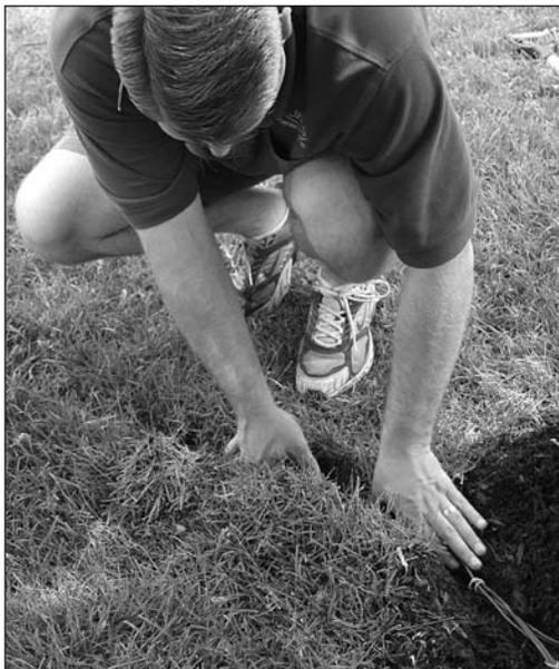
Wires are pushed firmly into the trench.
