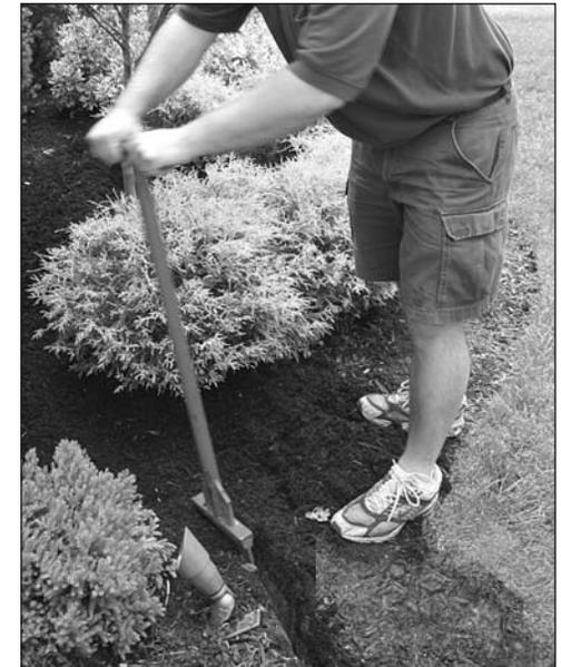
Pushing the tool back and forth widens the trench and creates a channel for the wire.
