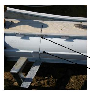
Step 10: CENTER ROLLING TUBE ASSEMBLY IS DONE AT TIME OF BLANKET INSTALLATION. Fit drive end and extension ends together tightly. Insert tee fasteners in holes at the side of the housing placing splice bracket over tee's on both sides. Place retaining clips on top and bottom of support legs.
