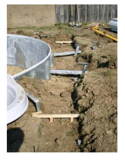
Step 9: You may now unpackage unit and place it in the prepared location. PLEASE ENSURE ARROWS ON TOP OF UNIT POINT TOWARDS POOL. DO NOT REMOVE LID PROTECTION UNTIL SOLAR BLANKET INSTALLATION. LID IS ALUMINUM AND WILL MARK IF IT COMES IN CONTACT WITH CONCRETE.
