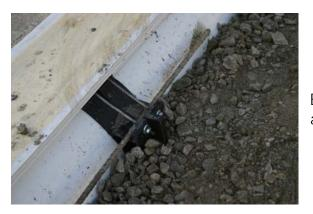
Backfill as usual and include the addition of some rebar for strength.
