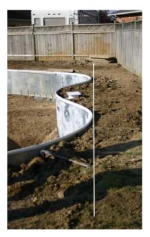
**Step 1:** To ensure the correct and square location of the Cleardeck run string lines on both sides of pool to properly align the Cleardeck unit with the outer most edges of the swimming pool surface.
