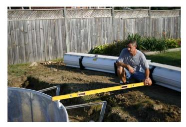
Step 4: Using a piece of coping installed on the pool wall and rebar, determine the elevation of the Cleardeck using a large level. Mark the level on the rebar.
