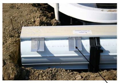
Anytime concrete does not reach under the top flange of the unit, install paver clips. The paver clips are longer and allow concrete to be poured lower down on the profile of the unit leaving space for stone to be laid right to the edge of the unit.
