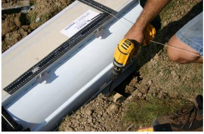
Step 12: Screw the unit through the bottom lip to the supports that you have created. This will ensure no movement of the unit will occur and you can now carefully backfill and cement in as usual.
