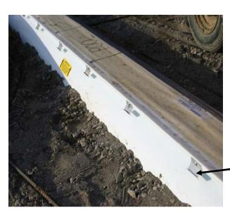
Install the concrete clips along the top edge of the unit. These clips will help bite into the concrete.
