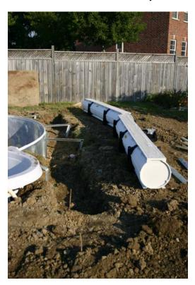
**Step 3**: Excavate an area of 20" wide to a depth of 20" where the Cleardeck will reside. Keep the unit as close to the pool as possible to reduce blanket wear. (Distance from coping can vary depending on the pool)
