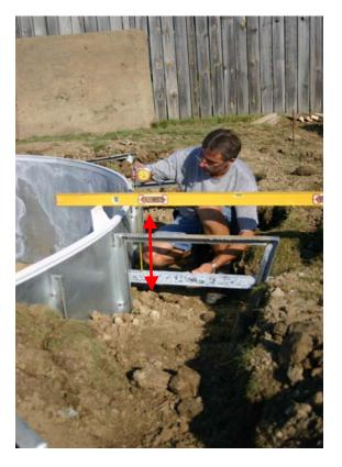
**Step 6:** Pool braces will need to be modified to create a space for the roller. Using a level, build supports the length of the Cleardeck. If the pool has no steel bracing, create a base to place the unit on out of lumber and stakes. (See Step 7)
