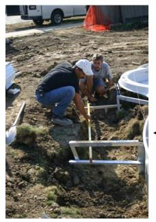
**Step 7:** Where the Cleardeck extends past the pool frames, construct a wood base to support each end of the Cleardeck unit. Please ensure that the wood braces are level with the supports attached to the deck frames and pool wall.
