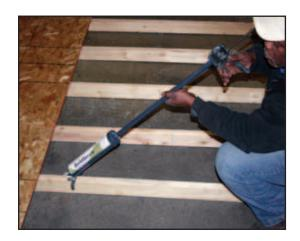
**BuildSecure** is a high-solids, solvent-free, no-odor, fast-setting polyether adhesive. **BuildSecure** is specially designed for bonding most construction materials including: wood studs, galvanized steel framing, aluminum framing, rafters, subfloors, drywall, gypsum, cove, fiberglass, FRP panels, ceiling systems and EIFS foam. It adheres to expanded polystyrene (EPS) and polyurethane foam.
