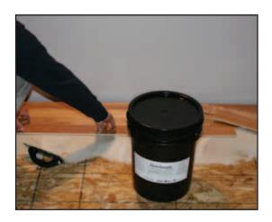
FloorSecure is a high-performance, polyether -based trowel grade adhesive for bonding wood flooring, tile and stone to most floor substrates. The nonflammable, high-solids formula is VOC-compliant, and its high initial tack, ease of application and greater adhesive coverage makes it the perfect choice for interior applications of most flooring materials.
