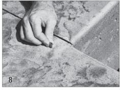
Insert plastic anchors (33)into the holes and tap with a hammer so they are flush with the deck. Fasten the lid to the deck with #12 pan head sheet metal screws (26).
