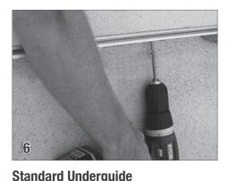
Clamp the guide with pulley to underside of the deck flush with the deck face. If water is in the pool, place the hammer drill with a 1/4" masonry (carbide-tipped) bit into a large bucket to drill holes approx. 3" deep on a slight angle toward the pool wall. Remove clamps and guides, then drive plastic anchors (33) into each hole. Finally, fasten the guides to the underside of the coping with #12 screws (26).
