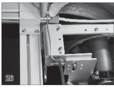
Run #8 copper bond wire from the lug on each guide feed to the lugs on each mechanism end.
