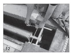
On the non-motor end, run the rope from the back channel of the guide around the pulley.
