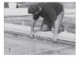
**Encapsulated Underguide (optional)** If encapsulation is being used, the guide is normally installed during the cover installation. (See cover installation section page 10, step 9).
