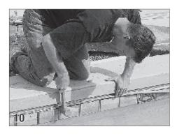
Insert and tap the spacer into place underneath the guide along the entire length of the guide. Do this along both sides of the pool. The spacer needs to end at the inside edge of the housing
