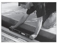
With the mechanism and tube assembled and set in place in the housing, check the roll-up tube for level. **This is crucial to proper operation of the cover.** Adjust height of non-motor end feet if needed to level the roll-up tube.
