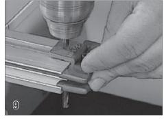
Holding the guide feed firmly, use a 6 inch 3/16"bit to drill through the hole in the guide feed and through the guide. Remove the guide feed. Do this for the guide on both sides of the pool.
