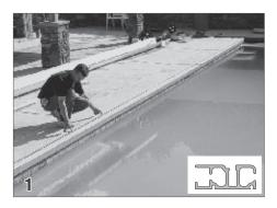
Lay the guide (14) on the deck on both sides of the pool.
