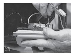
Insert the hot wire from the power supply into terminal L1 on the back of the switch and tighten the screw. Do not loosen the screws too much or the internal switch connections will be permantently lost.
