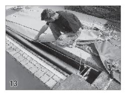
Pull the rope along the back of the housing to the motor side.
