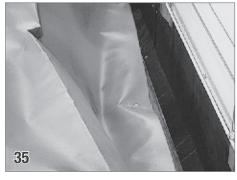
The first two screws need to be 3" from the end of the tube. Distribute the slack of the cover evenly across the length of the tube. Secure the cover to the roll-up tube using tek screws (32) every 2-3ft. When attaching the cover to the tube, **do not use folds or pleats**.
