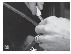
Connect the ground wires from the power supply and the motor together using a wire nut. Run a pig tail from this wire nut to the grounding lug on the switch.
