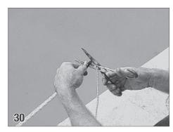
Pulling both ropes tight, cut the longer rope to the same length as the shorter rope. These ropes should be at least 8ft long. Use a lighter or torch to burn the ends of the rope. In most cases you will only need to cut one rope.
