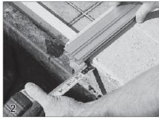
Cut the guide so it will extend from the front edge of the coping at the far end of the pool to 1" inside the housing.
