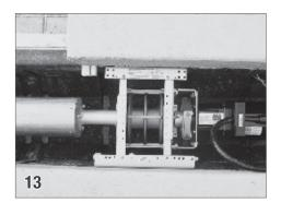
Raise the pulley brackets up so that the top of the bracket is even with the top of the encapsulation or guide. This insures the ropes will be level.
