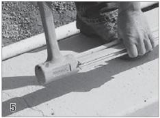
Lay the sections of guide on the deck and tap them together using a rubber mallet so the splice and pins interlock with each section of guide. It's important that, the splice is tight together so there is not a gap from one guide to the next. Slide pulley end cap (15) into the end of the guide.
