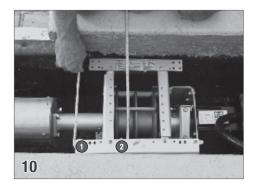
Align the mechanism on the motor side first by using a straight edge or a piece of rope and extending it from the back side of the cover guide to the pulley to make sure the rope is running straight into pulley #1. **Tip:** 2 Pulley bracket should be 1 inch from outside of guide.
