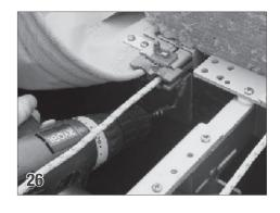
Secure the guide retainer to the wall of the housing using 1 1/2" hex head screws and anchors. Install the guide feed and retainer on the other side of the pool.
