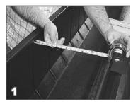
Check the inside width of the cover housing. Make sure it matches the width of the flush lid kit that was ordered.
