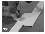
Slide the two sections of lid together. Slide the descenders on the front side of the lid. Position the lid in so it rests on the lip of the riser and on the lid brackets. Make sure the lid is in place when the concrete is poured. The lid can be masked off or turned upside down to keep it clean during the concrete pour.
