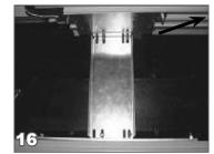
Install the cross braces over the pem studs in the *QuickAttach* brackets at both the motor and non motor ends of the housing. These cross braces will maintain the correct width between the *QuickAttach* mechanism mounting plates during the concrete pour. Secure using ½ - 20 nylock nuts. These cross braces will be removed when the mechanism is installed.
