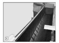
Measure across the back of the housing between the boxed ends. Cut a length of the riser (X0944) to fit in this opening.
