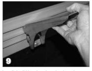
Install the lid brackets into the riser along the back of the housing. Place a level on the brackets and level them by adjusting the bolt at the bottom of the bracket.
