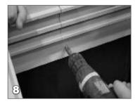
Secure the riser to the housing by screwing 1 inch self tapping screws (H9614) through the riser and into the housing. Make sure the top of the riser is flush with what will be the finished deck height.
