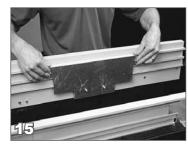
Insert the *QuickAttach* mounting plate over the appropriate anchor plate.
