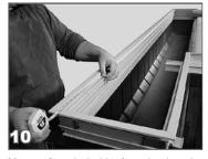
Measure from the inside of one riser boxed end to the other in order to determine the total lid length. Cut the lid panels to this length.
