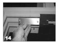
Position the anchor plate into the top channel of the riser by inserting it at an angle so the top of the anchor plate goes into the channel first, and then move the bottom of the plate into the channel. Repeat this process for the other anchor plates.
