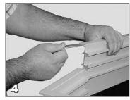
Insert splices (M9351) in the splice channel of the riser so they will extend part way into the splice channel of the of the riser and hox end.
