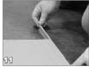
If a lid descender is being used, cut the descender to fit across the front of the lid between the coping. Also, cut the flat no profile descender to fit on the motor and non motor ends of the lid. If a profile descender is not being used, use the flat no profile descender (A1752) across the entire lid.
