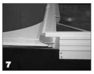
If using a Coverstar Encapsulation with coping, install the transition pieces that will fit between the riser panel and the encapsulation/coping.
