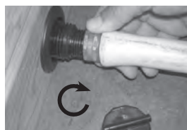
3. Thread hose onto the spa drain
