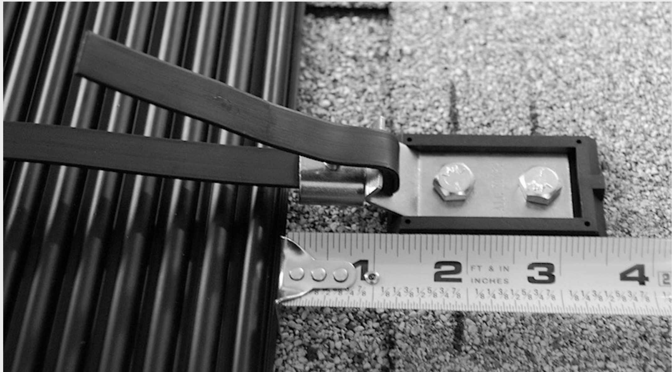
FIGURE 7 Termination Strap Bracket Assembly
