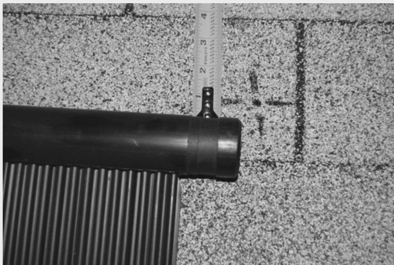
FIGURE 3 Outlet Header Bracket Location
