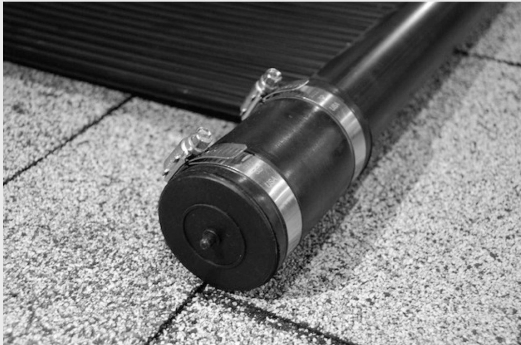
FIGURE 11 Installed End Cap
