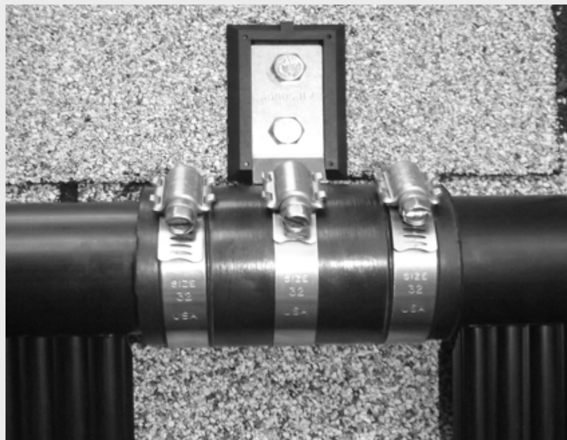
FIGURE 5 Installed Outlet Header Bracket with Hose
