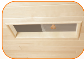
Sliding Roof Vent
