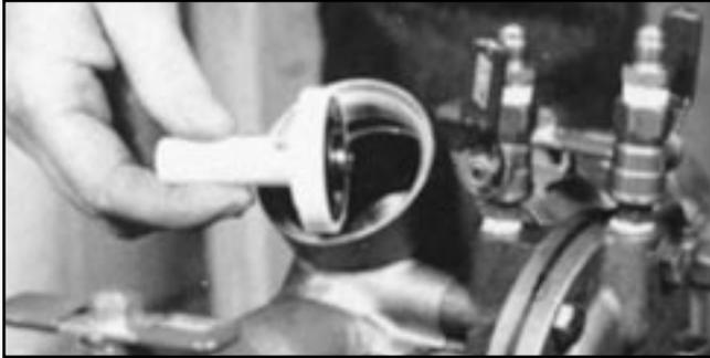
The line should be flushed clean of debris before installation of the assembly. To flush the line after installation of the assembly, slowly close the inlet shut-off valve, remove the covers and internal assemblies of both check valves and open the inlet shut-off valve to allow sufficient flow of water through the assembly to clear all sand, debris, etc. from the line. If debris in the water continues to cause fouling, a strainer may be installed upstream of the assembly.
