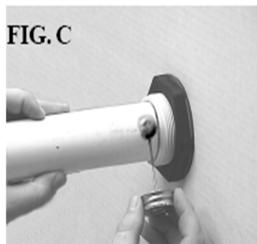
This lens assembly should glue directly on 1 1/2" PVC pipe. DO NOT GLUE A REDUCER BUSHING DIRECTLY INTO THE LENS HOUSING! If you want to reduce to 1" PVC pipe, do so with a reducer after a few inches of 1 1/2" PVC pipe. This is to allow room for the lens assembly to seat into the body of the lens housing. The LNS-2A must be installed 12" to 14" down from top of wall.
