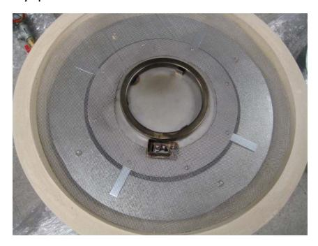
Lay down precut stainless wire screen over Grand Effects Burner Assembly. Make sure that the Grand Effects Burner Assembly is using the Pilot Box Cover option as shown above.
