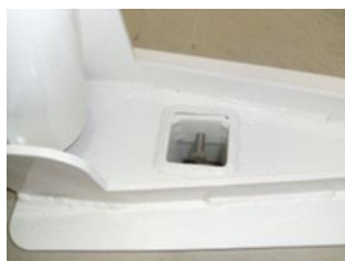
3/8" bolt inside anchor sleeve
