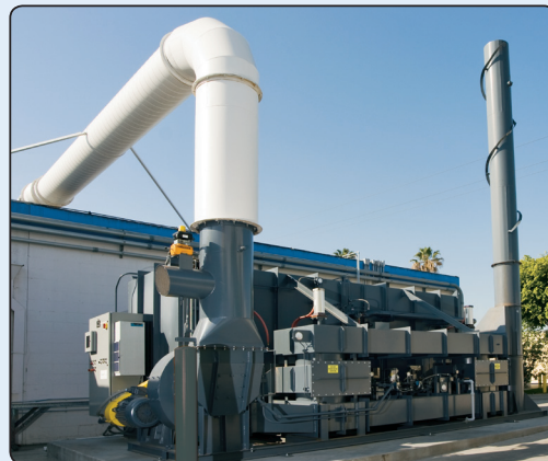
Our California facility takes pride in limiting volatile organic compound (VOC) emissions into the environment. Two regenerative thermo oxidizers are utilized to eliminate 99% of the VOC from our ventilation system before emitting air to the atmosphere.
