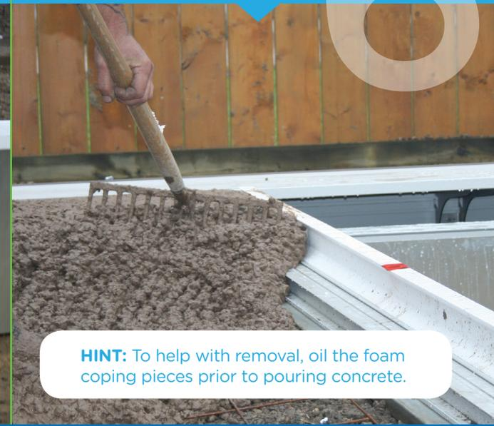
**HINT:** To help with removal, oil the foam coping pieces prior to pouring concrete.
