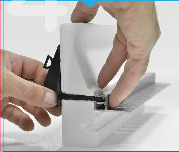
When installing the next 8' piece, ensure pieces are tight together and tape over the joint.
