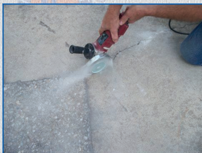
Rout crack with crack chasing blade or regular diamond blade.
