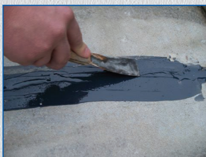
Immediately spread dispensed Speed Bond into crack and onto adjacent sides of slab with putty knife.
