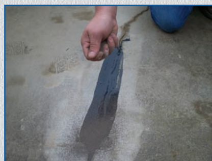
While Speed Bond is still wet evenly broadcast silica sand over it and allow to cure. Once cured, brush away any remaining sand residue. The crack is now ready to be coated.
