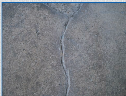
Thoroughly clean crack of all dust and debris.
