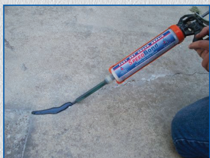
Place tip into bottom of crack, dispense material and slightly over fill. Do not allow material to set in tip for longer than 1 minute.
