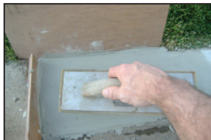
TROWEL OUT LEVEL WITH ADJACENT SURFACE.
