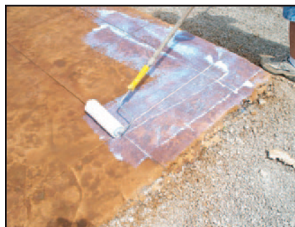
AS SOON AS MULTI-STAIN HAS DRIED, USUALLY THE NEXT DAY, APPLY 2 COATS OF MULTICOAT'S CLEAR SEAL TO LOCK IN THE COLOR AND PROTECT THE SURFACE.
