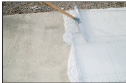
MIX STAMP MIX WITH WATER, APPLY TO 1/4" THICK WITH GAUGE RAKE.
