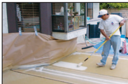
APPLY DILUTED FIRST COAT OF DECK PAINT WITH ROLLER
