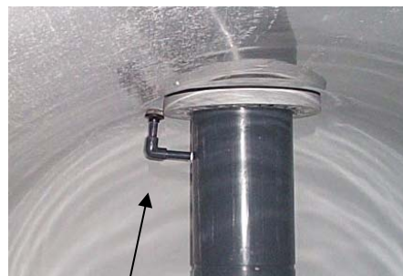
Automatic Air Relief Assembly
