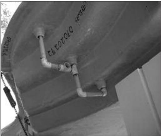
Plumbing the Vantage system while on the delivery trailer (if the driver can wait) or on the ground before setting, makes the job easier. (if you must set your pool on the ground, be sure to place support blocks under it, do not allow the pool to rest on Vantage ports.)
