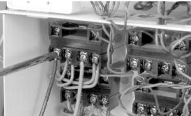
Fig. 6B – Wiring connections to be made inside time clock or electrical panel.
