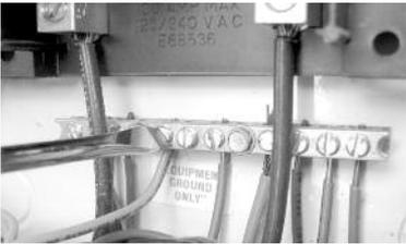
Fig. 6A – Wiring connections to be made inside time clock or electrical panel.
