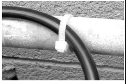
5. Lay the 3/8 tubing along desired route to the compression fitting on the combination needle valve flow meter on the Clear O3® unit.
