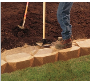
2. Place & Compact Backfill
