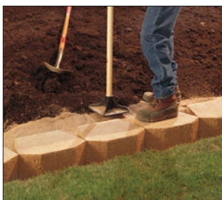
2. Place & Compact Backfill
