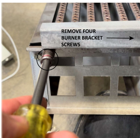
Figure 2. Remove Four Burner Bracket Screws
