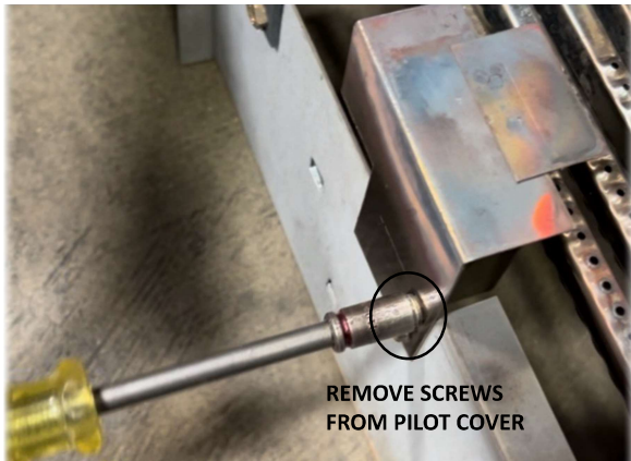
Figure 6. Remove Pilot Cover Screws
