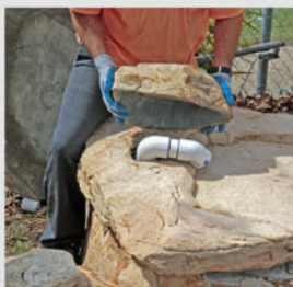
6" plumbing sleeve for 2" pipe should be filled with spray foam or mortar after pipe is set
