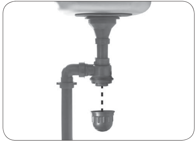
Fig. 4-1 Drain trap cleaning
