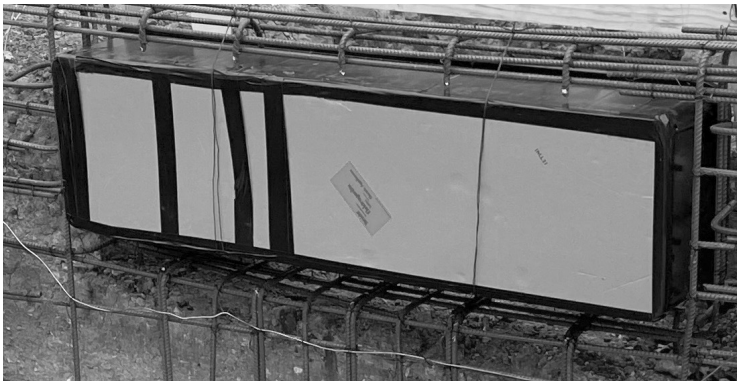
Image 4 BADUJET Turbo - Jet placement in rebar
