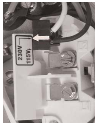
Figure 5A -Voltage Change Plug Set for 230 Volts
