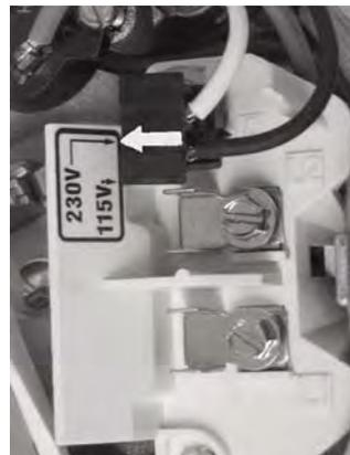
Figure 4A -Voltage Change Plug Set for 230 Volts
