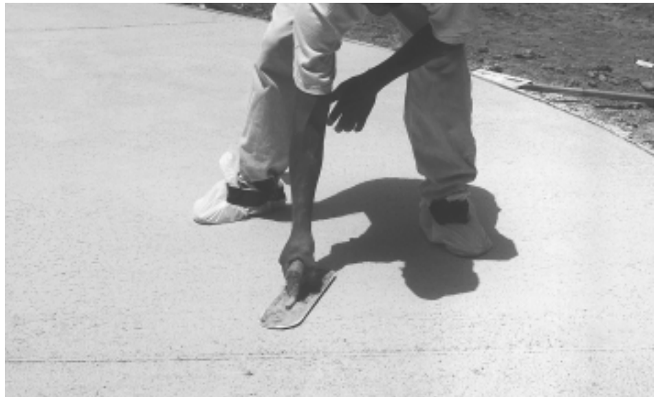
Soft plastic bags allow the finisher to apply the final pass without leaving foot prints.
