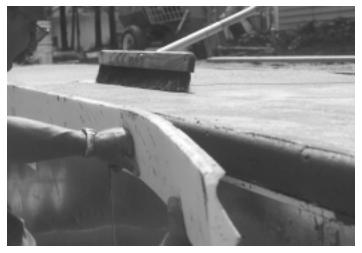
3. The cantilever form should be stripped at approx. the same time the brooming process is taking place.
