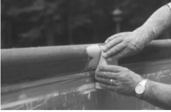
4. In the event that patching is required, use a small amount of the FDD material. This material should be taken from the mixer before the final wetting-up process. The Foam Profile Edging Tools are available to match each Stegmeier deck form profile.
