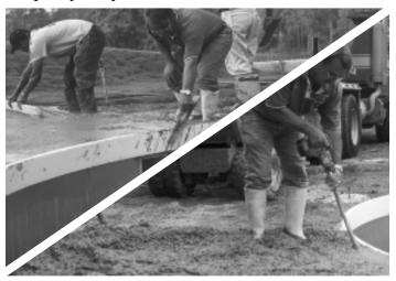
2. While pouring the base slab, care should be taken to pat or vibrate the cantilever form well, ensuring against rock pockets (honey comb). Place and finish concrete as previously described.
