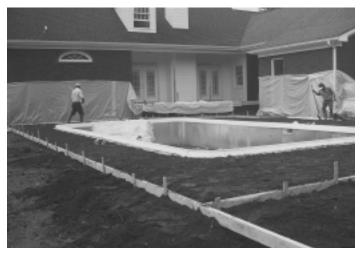
1. Whether the cantilever forms are set the day before or the morning of the pour, care should be taken to be completely ready when the concrete truck arrives.
