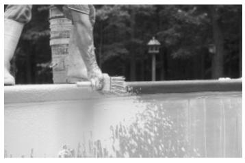
5. The cantilever edge should be dashed one section at a time, just prior to dashing the top slab.
